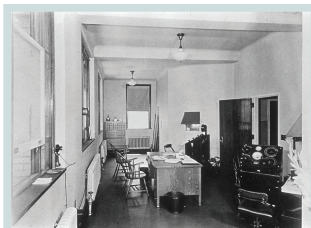
Figure 2. The First X-Ray Treatment Room
